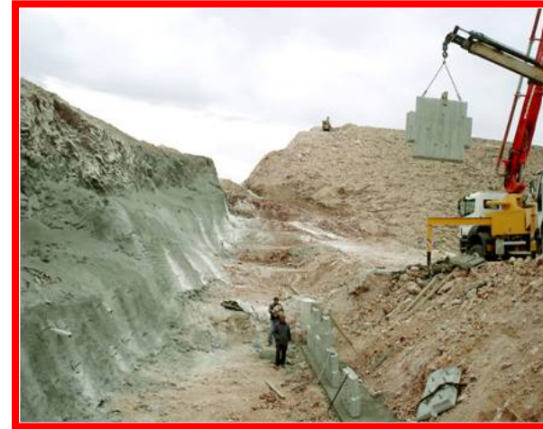
Erection of the first row panel
