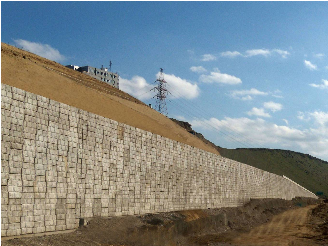
Baku bypass highway (Azerbaijan)
