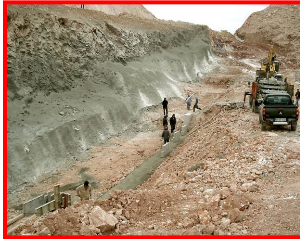
Erection of the first row panel
