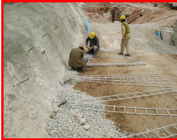
Secondary Reinforcements (Ladders) strips are connected to soil nail heads
