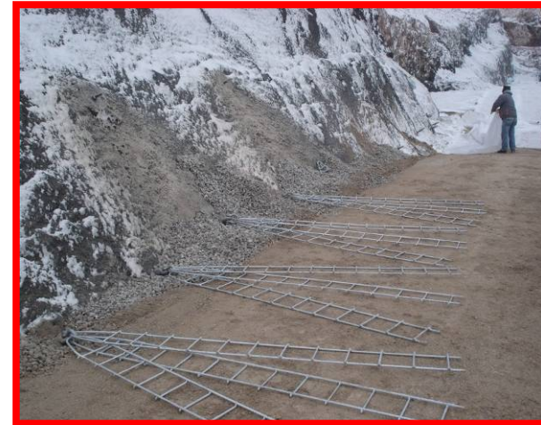
Secondary Reinforcements (Ladders) are connected to soil nail heads
