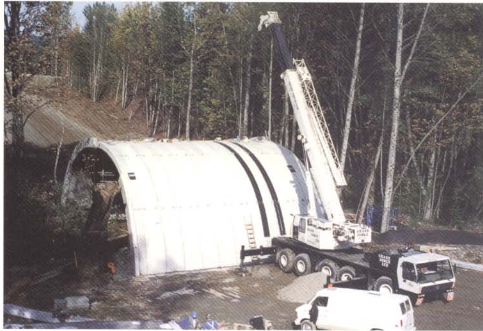
👂 Joints can be covered with geomembrane or geotextile. Optionally the entire arch can be waterproofed.
