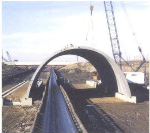
During TechSpan erection conveyor activity continues.
