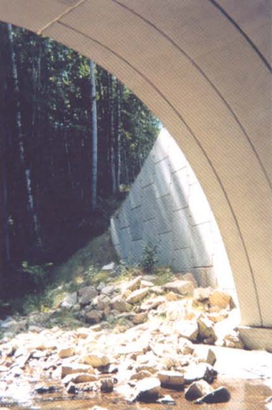
Environmentally sensitive creeks spanned without disturbance.
