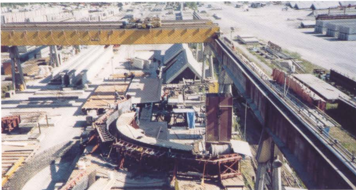
Reinforced Earth's engineered forms are used to precast TechSpan panels.
