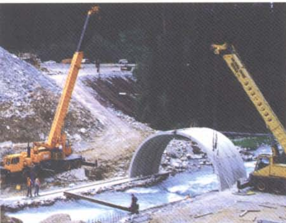
🎧 A short TechSpan of 20 meters length is completed in 2 days.
