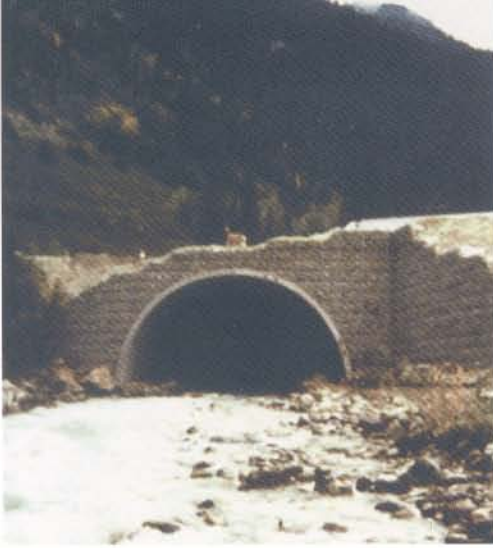
🎧 Terratrel collar wall with rock fill.
