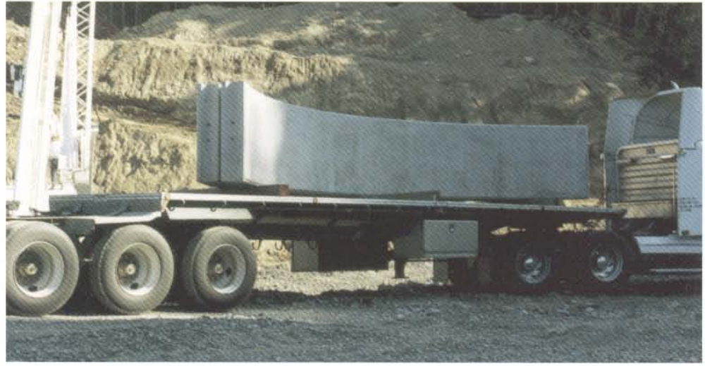
Elements can be installed directly from truck with timely coordinated deliveries.
