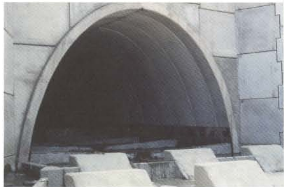
TechSpan culvert accommodates channelized flow.
