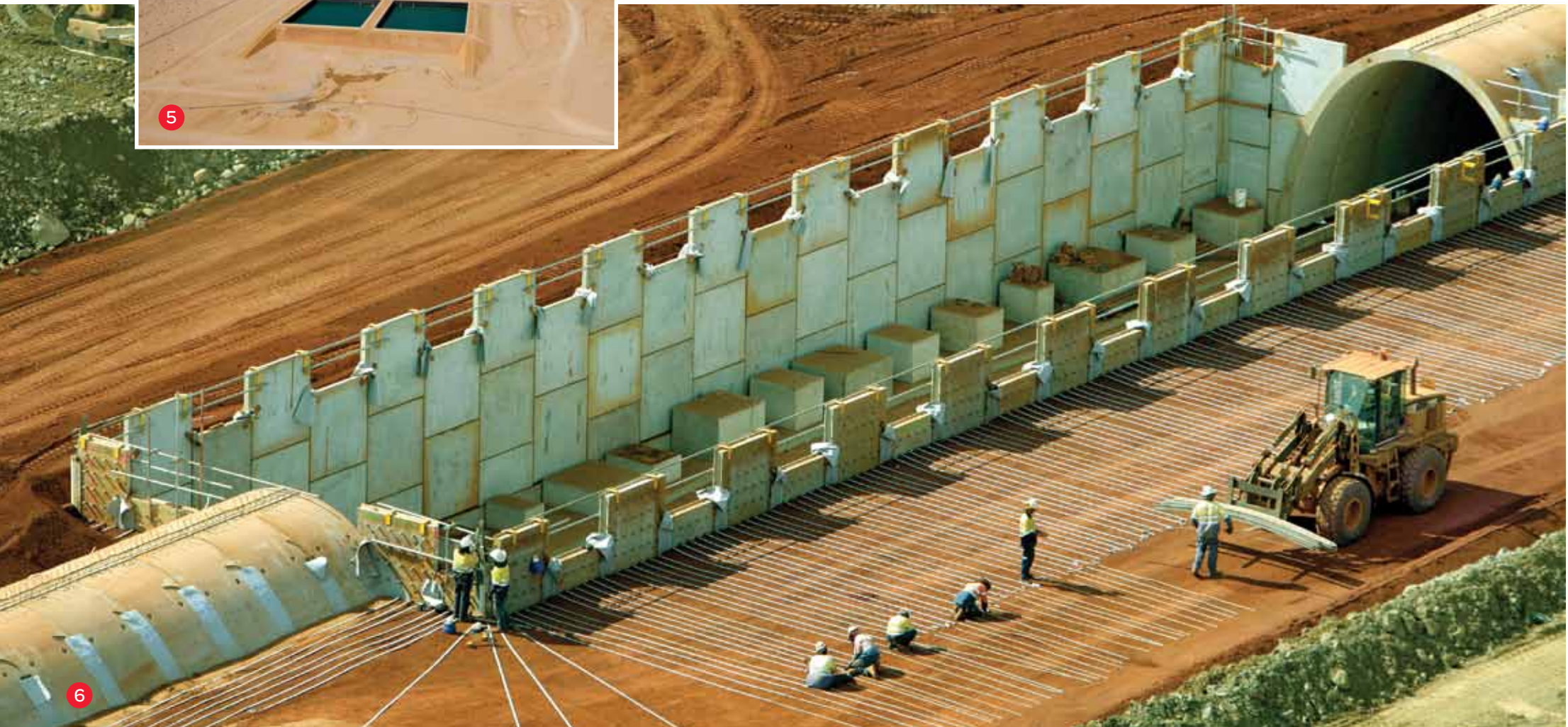
6. Iron Ore Mine / Western Australia Reinforced Earth™ vault and TechSpan® reclaim tunnels
