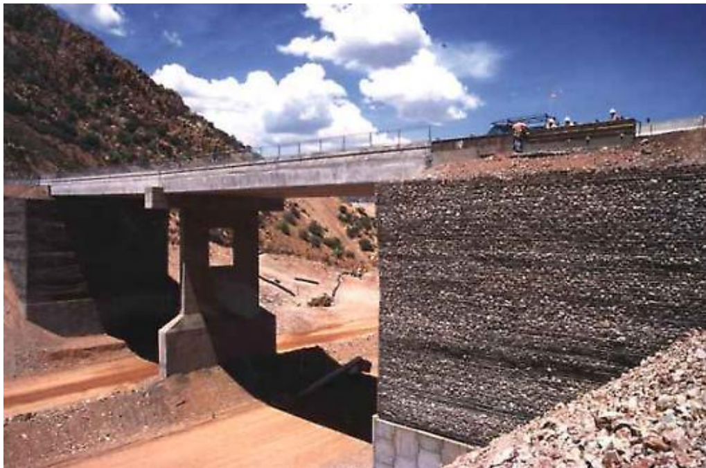
Morenci Mine Haul Road – USA (Reinforced Earth® and GeoTrel®)
