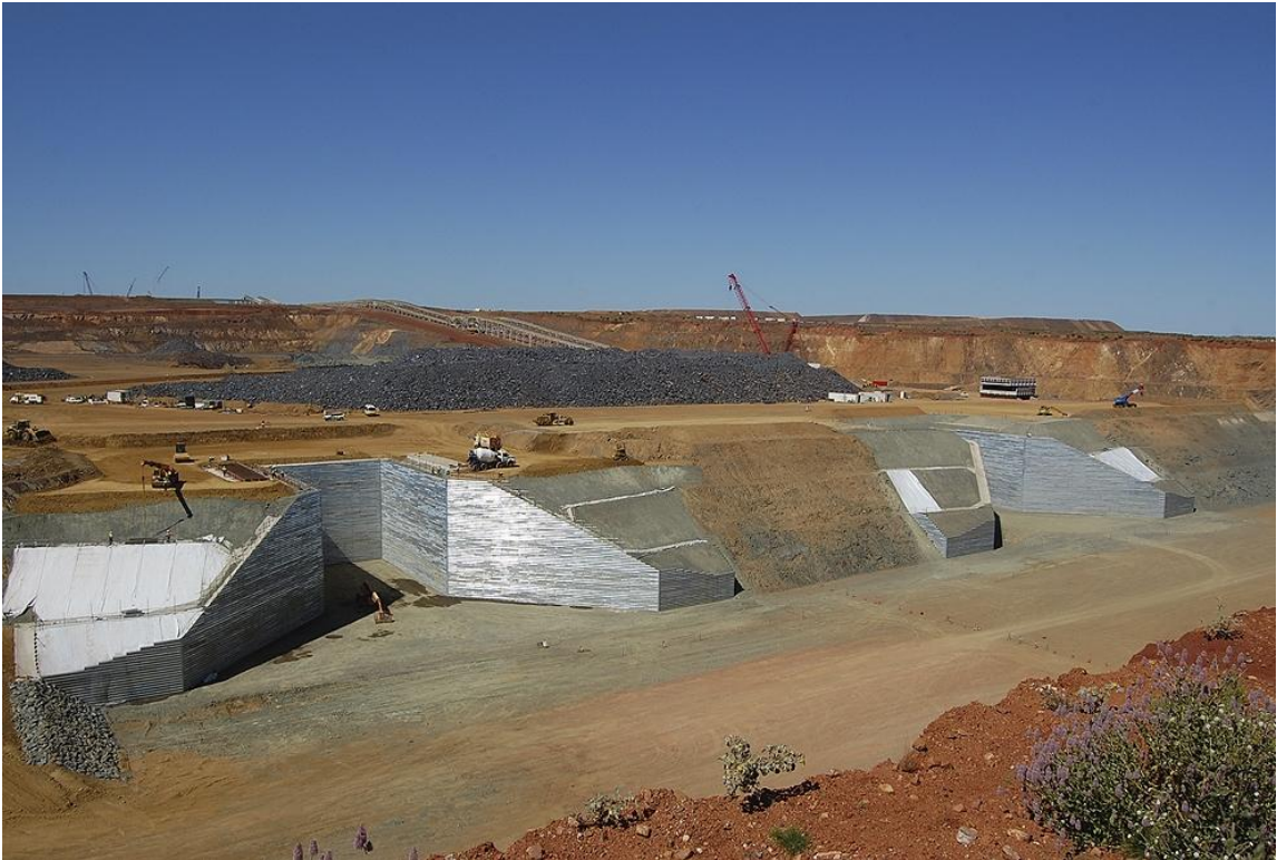
Sino Iron Project, Cape Preston, Australia (Reinforced Earth®)
