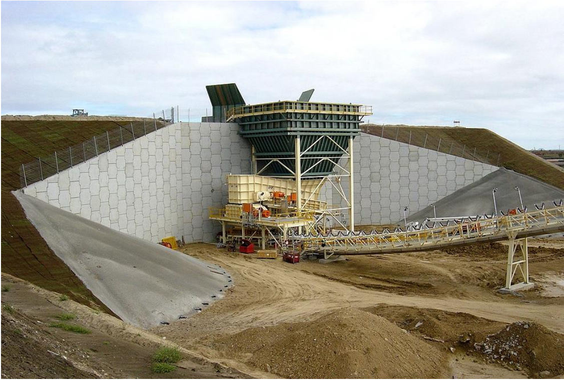
Rolleston Dump Wall, Central Queensland, Australia (Reinforced Earth®)
