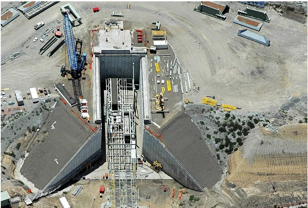
Blackwater CHPP Project, Central Queensland, Australia (Reinforced Earth®)
