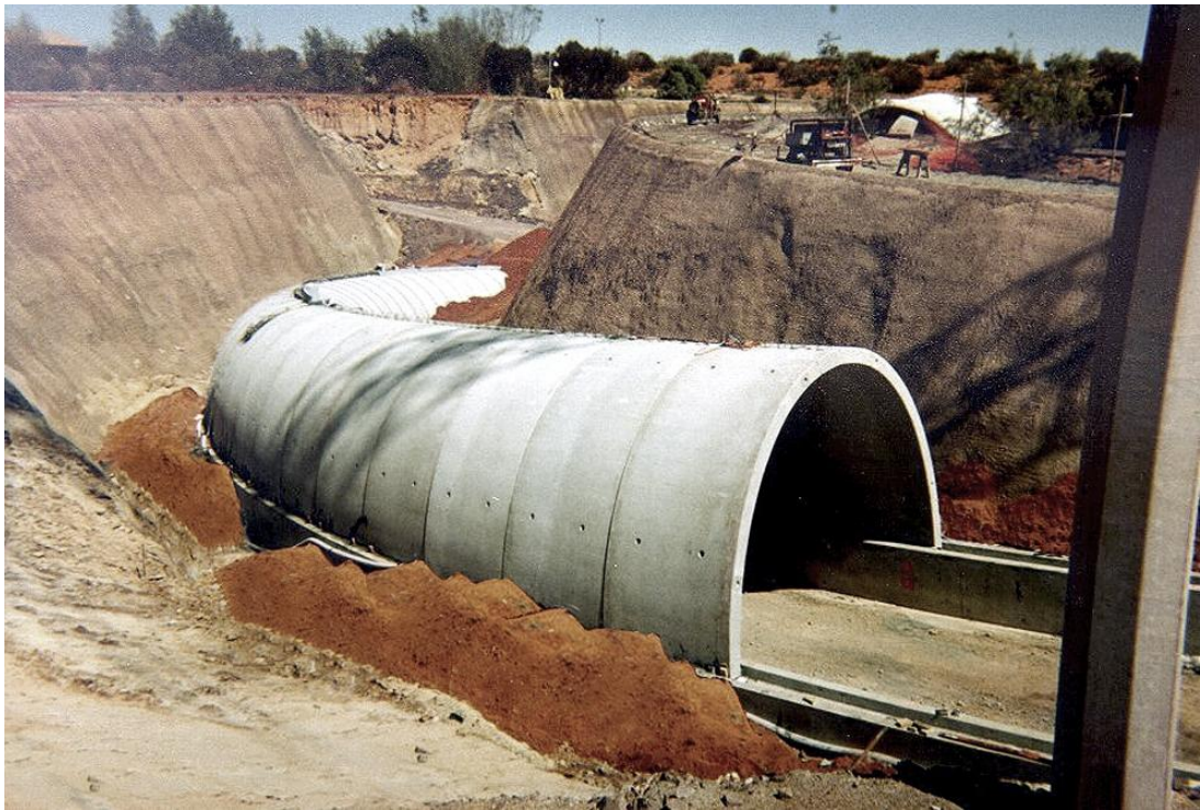
Tunnel, Olympic Dam Mine, South Australia (TechSpan®)
