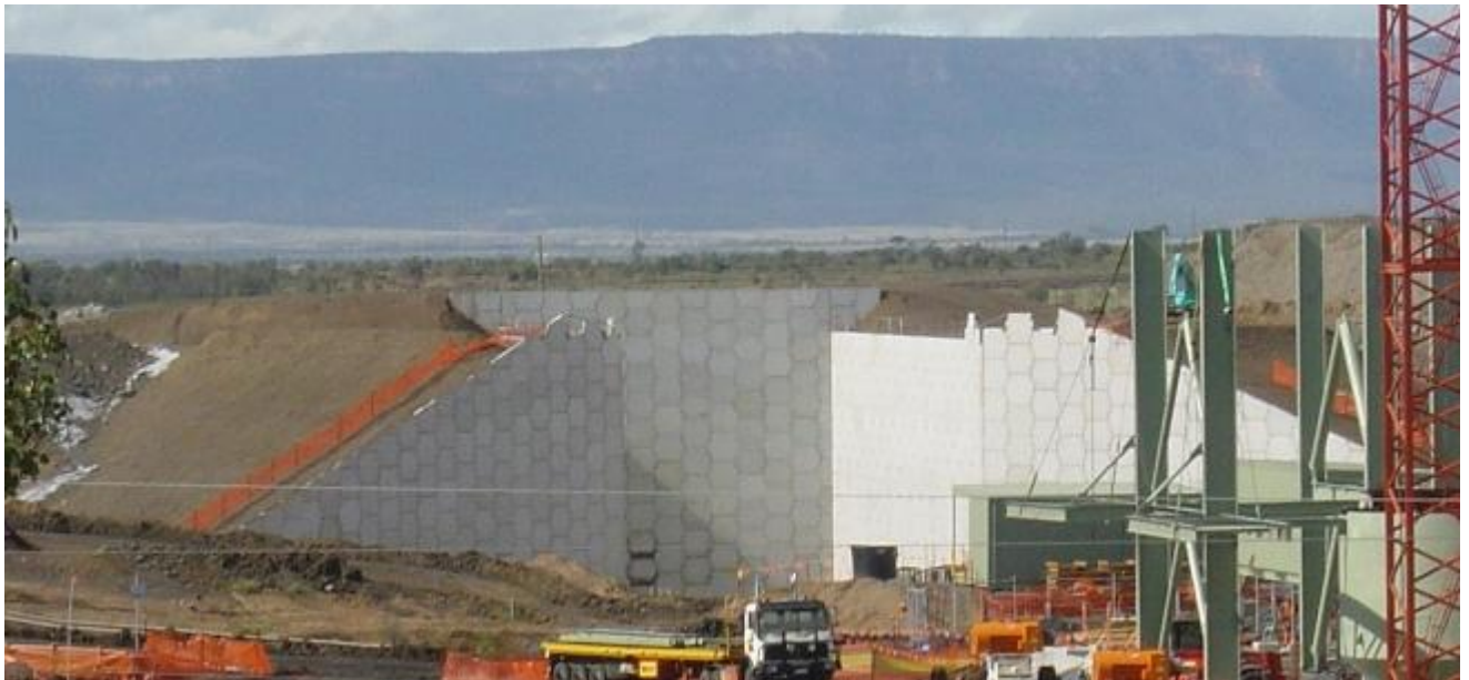
Cloud Break Mine, Pilbara, Australia (Reinforced Earth®)
