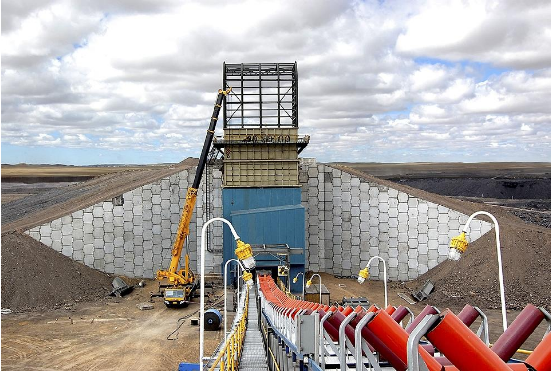
UHG Coal Handling Preparation Plant, Mongolia (Reinforced Earth®)
