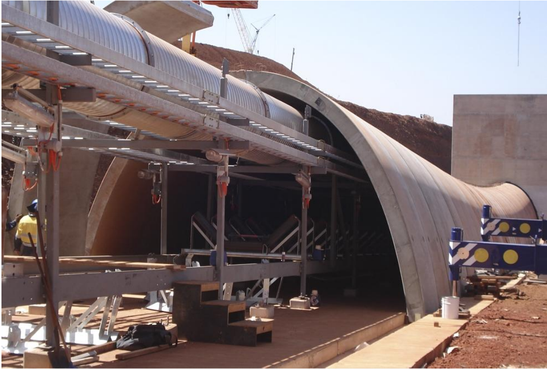
Cloud Break Mine Reclaim Tunnel, Pilbara, Australia (TechSpan®)
