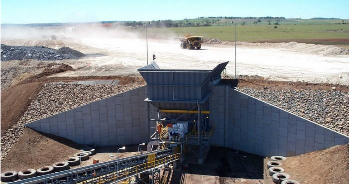
Poland (Reinforced Earth®)
