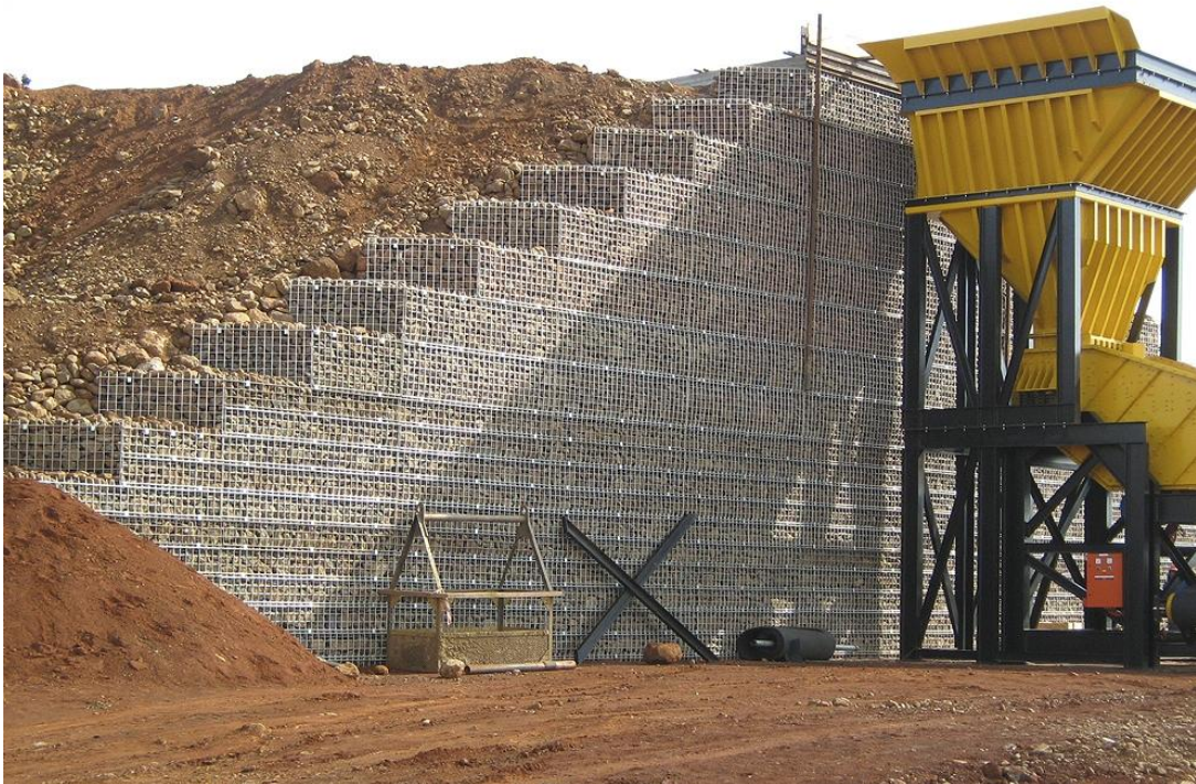
Bleugum Mine, South Africa (GeoTrel®)
