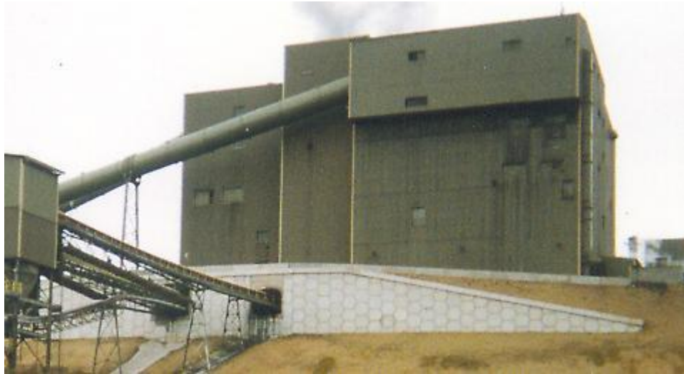
Prep Plant Headwall - USA (Reinforced Earth®)
