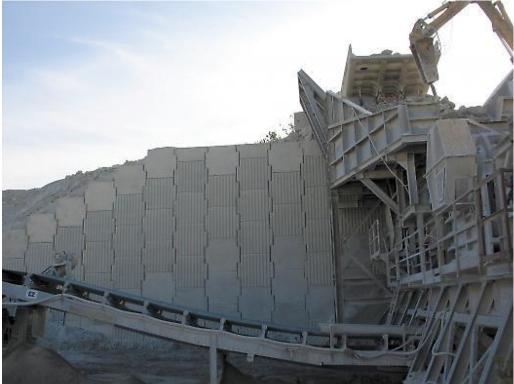
Plainfield Quarry, IL - USA (Reinforced Earth®)
