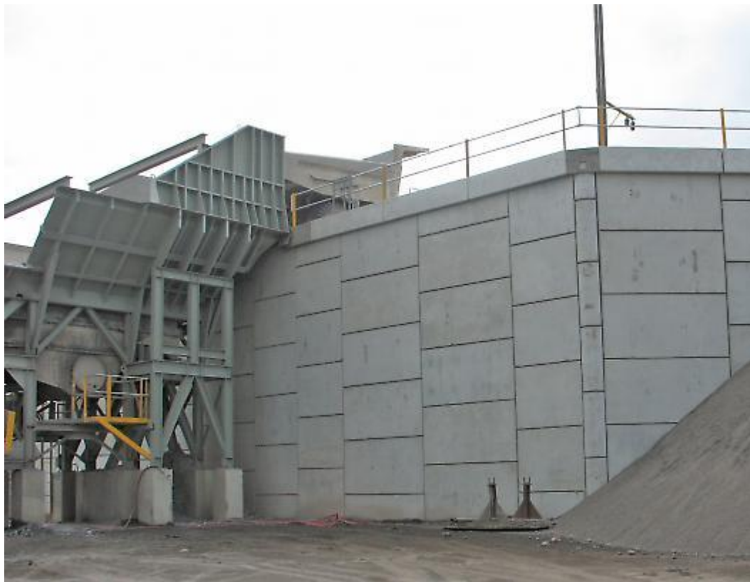
Crusher Unit - USA (Reinforced Earth®)
